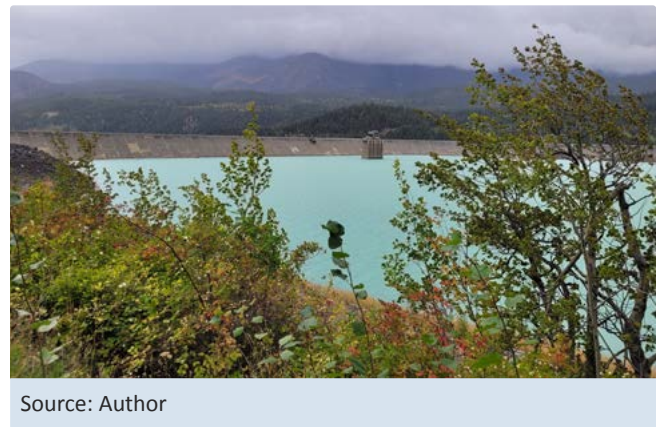
Figure 11: Lajoie Hydro-Electric Dam & Generating Station near the Reliance Project
