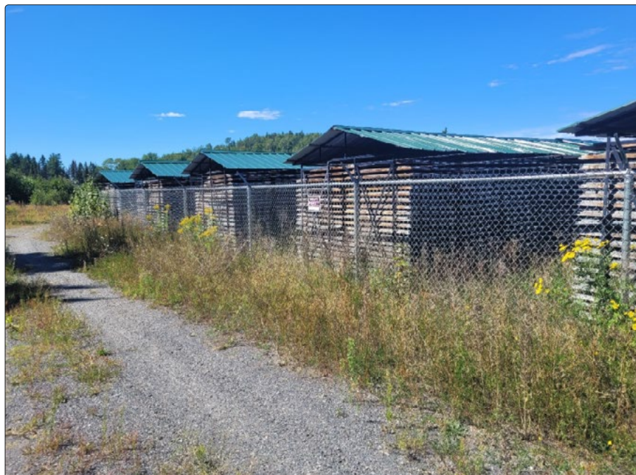
Photo 4: Secure core storage
