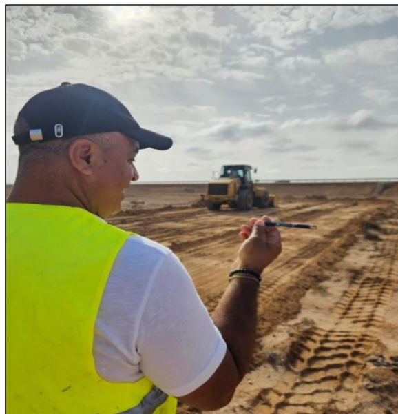
Figure 3: Facing East at the TitanBeach Project (Source: Company Documents)
