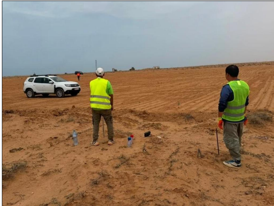
Figure 2: Preparatory Work for the TitanBeach Project Pilot Plant (Source: Company Documents)
